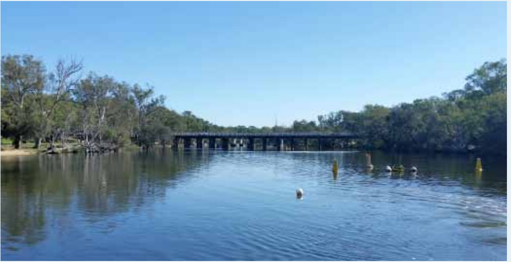
The Swan river, with Bassendean Bridge in the distance. A monitoring station (indicated by the buoys) tracks the levels of dissolved oxygen in the water and triggers the plant to turn on and off.
