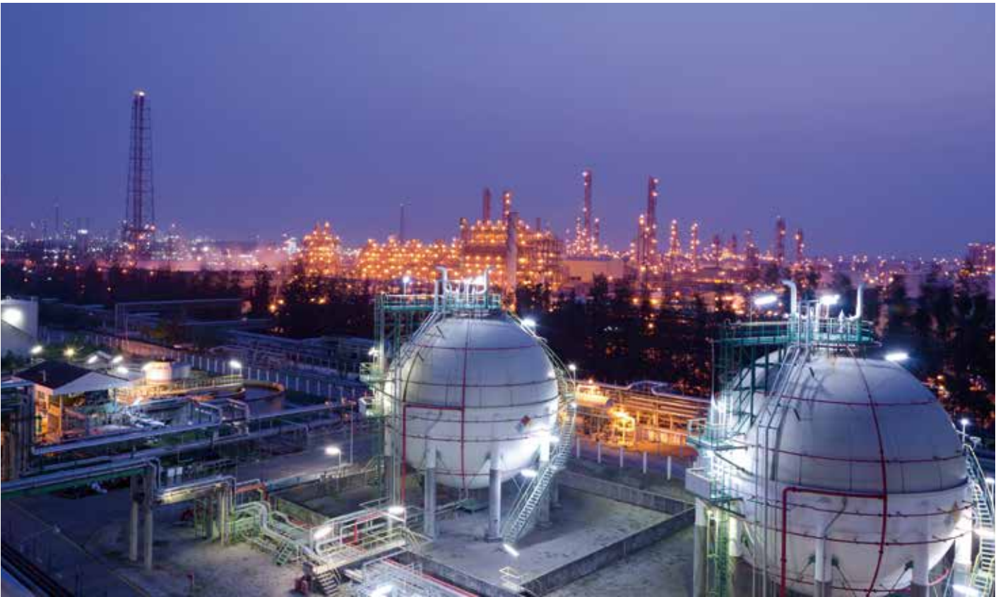
Oil refinery storage tanks
