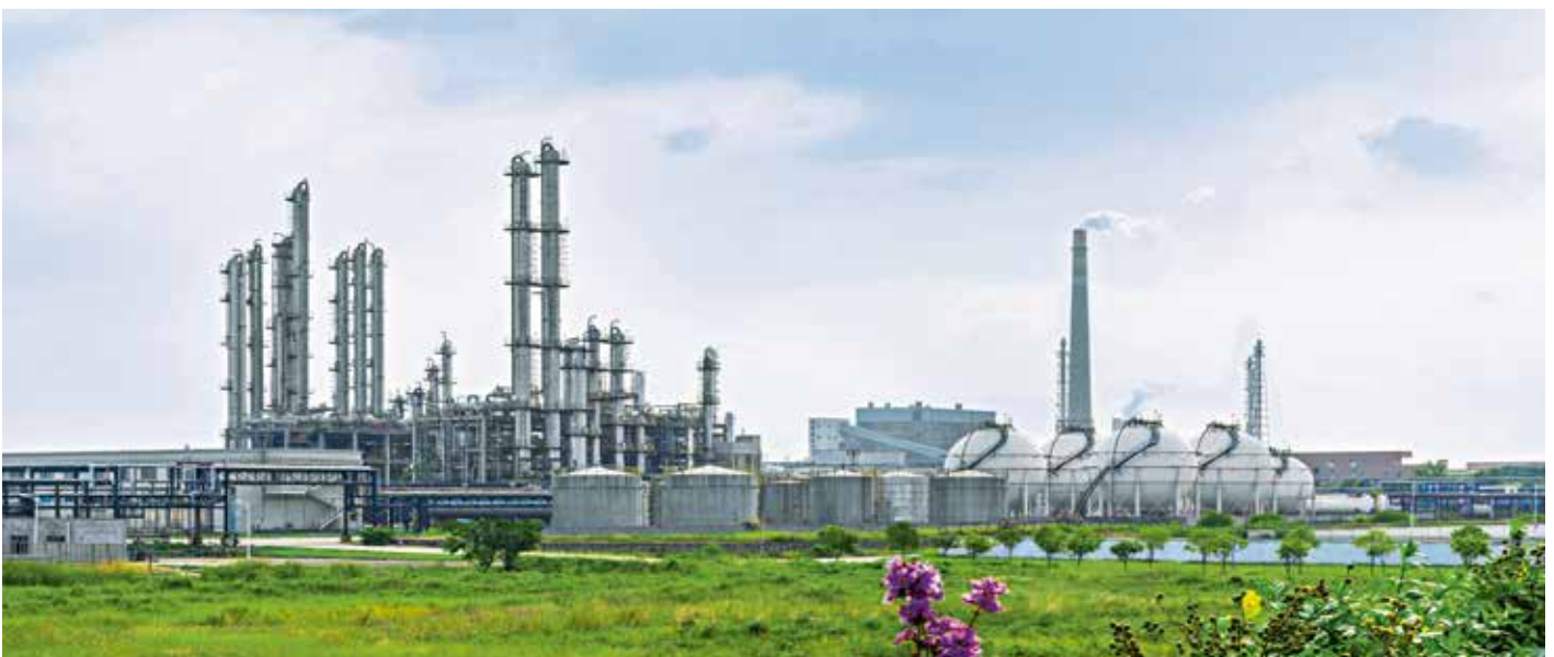
Refinery and its storage tanks
