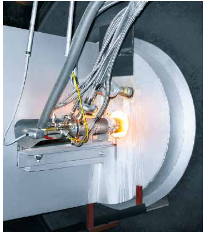
WASTOX combustion process and an oxyfuel burner in a double-pass furnace at Kuusakoski Oy, Finland.
