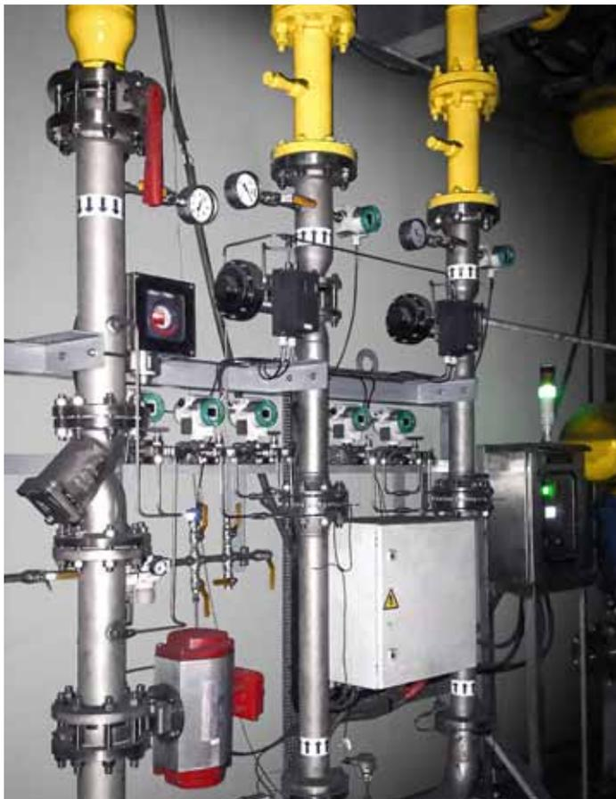
The oxygen flow control panel, controlling the flow of oxygen into the furnace.
