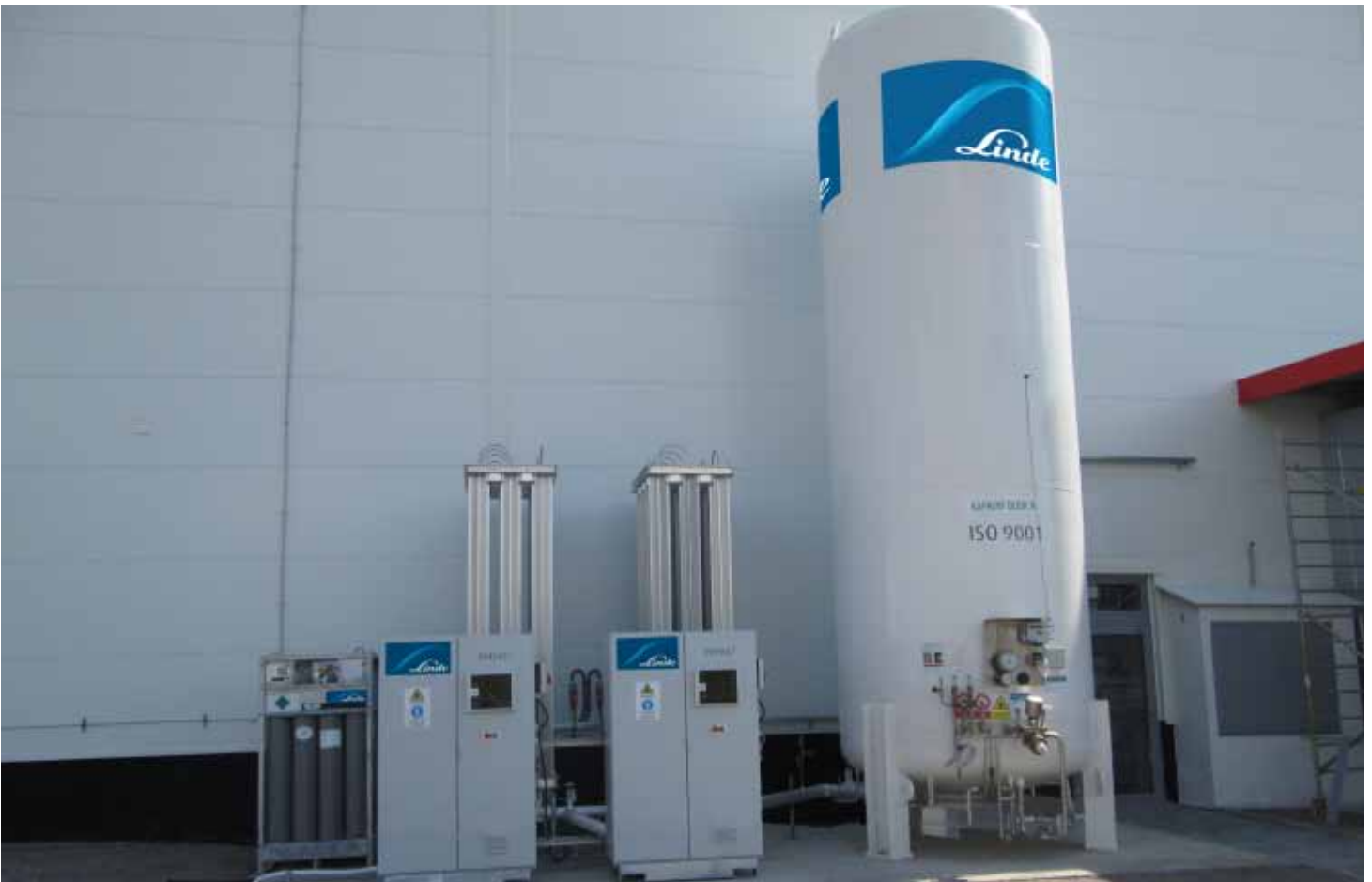
The centrepiece of the PLASTINUM® Gas Injection Moulding technology in Ostrov: the PRESUS® N10 pressure booster, which is supplied with liquid nitrogen from a tank. (Source: Linde)
